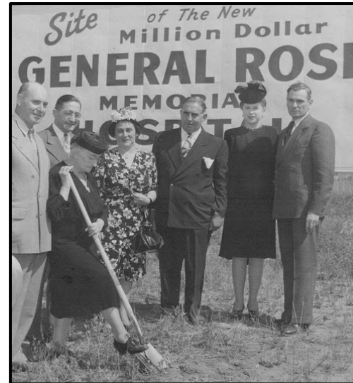
Mother, Katy Rose, breaking ground on the General Rose Hospital in Denver
