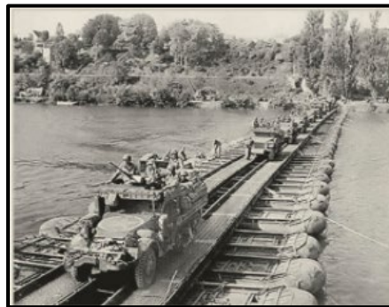
Tanks cross pontoon bridge built by unit under Gen Rose command.
